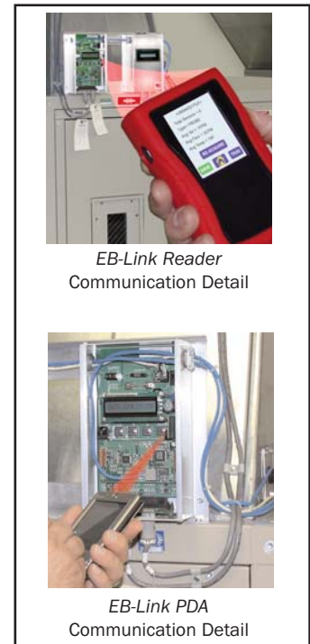
Figure 14. Typical EB-Link Data Acquisition
