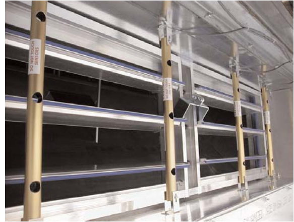
Figure 8. Typical OA Damper Installation
